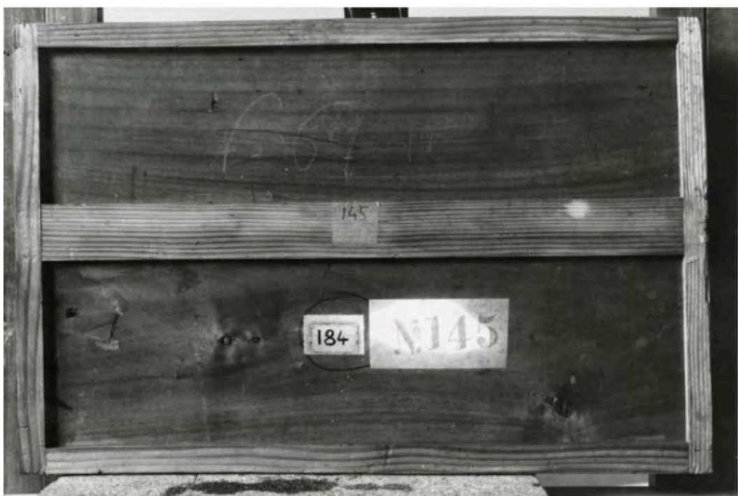
Archive photo of the framing prior to the 1972–73 intervention
