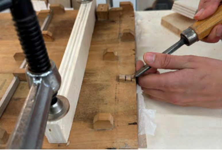
Photo 5 - Removal of previous parquetry
