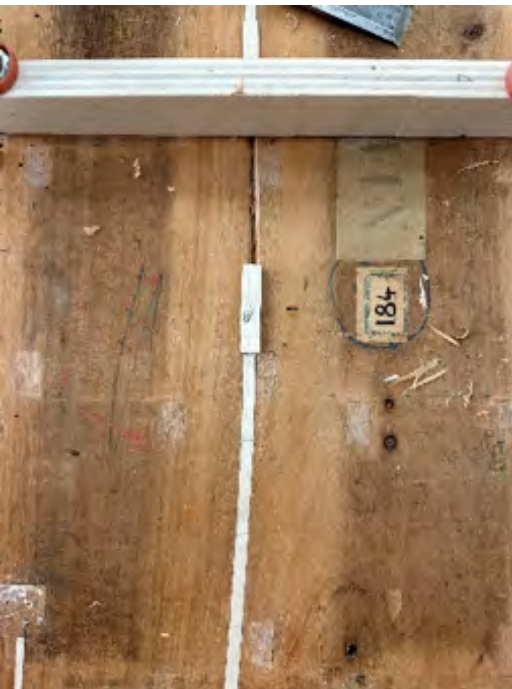
Photo 7 - Replacing the previous restoration
